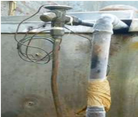
Fig-3 Capillary tube
